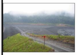
The Rocklick Branch Refuse Impoundment is a coal slurry refuse dam. The dam is a class C hazard dam and is located on Rocklick Branch of Pond Fork, located 1 mile upstream of Greenwood, in Boone County, WV. The coal refuse impoundment is built using upstream construction and is classified as having high hazard potential. The dam is approximately 470 feet high, measured from the downstream toe, with a 110-foot wide crest at an approximate elevation of 1,670 feet above sea level.
